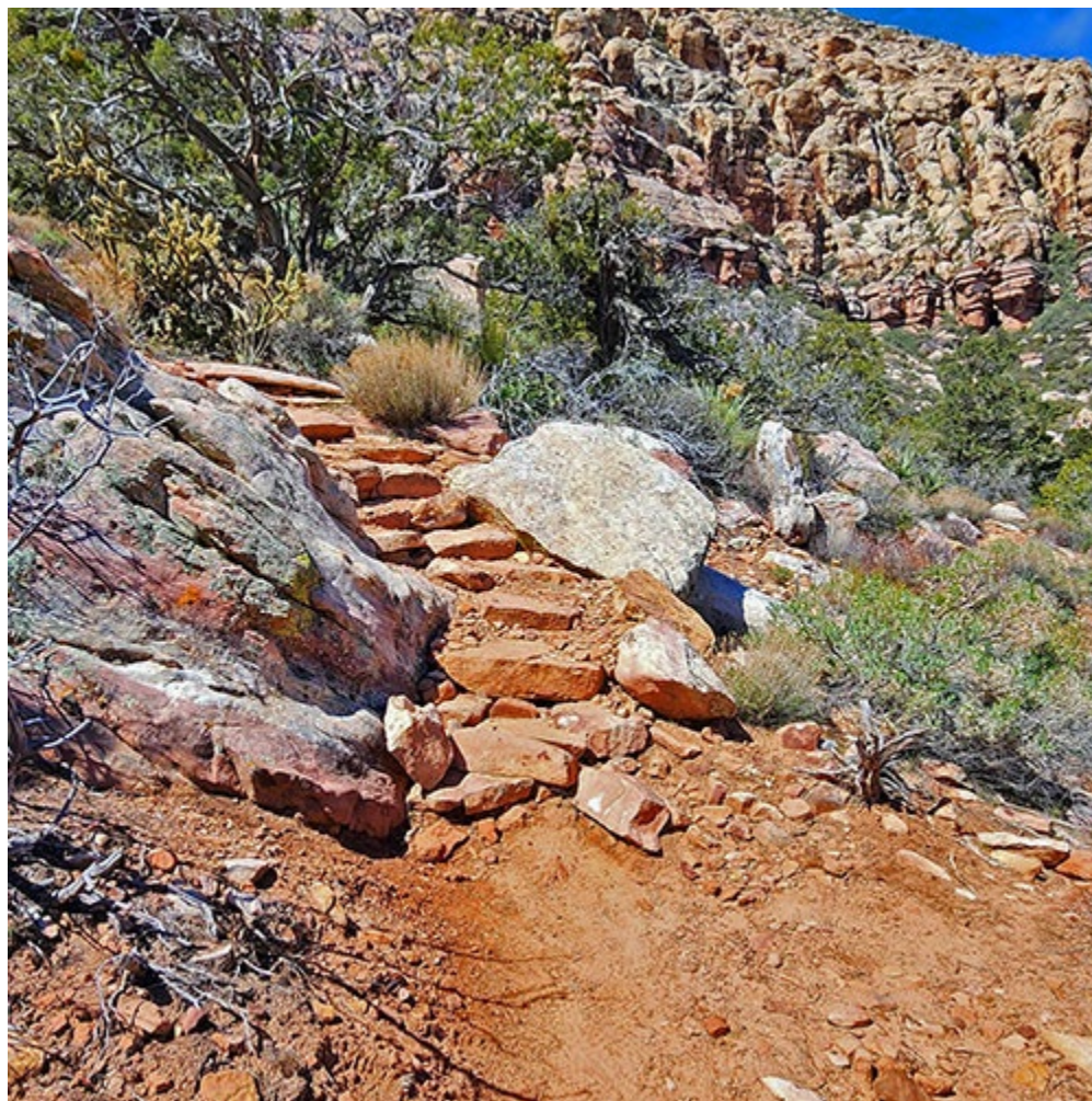
Artistically Constructed Stairway on The SMYC Trail
